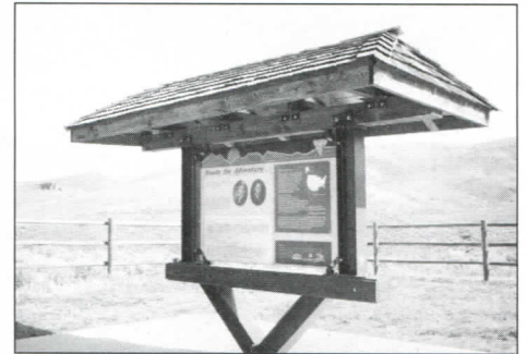
The Bureau of Land Management is constructing several new Lewis and Clark interpretive kiosks—such as this one on the way to Lemhi Pass.
