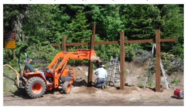
**Canyon Junction sign reconstruction.** Dick Monaghan with his tractor lifts a post for placement. Carl Stone and Geoff Billing guide the post into the hole. The posts are 8x8 inch by 12 feet long w4x6 cross piece that carries the signs.
