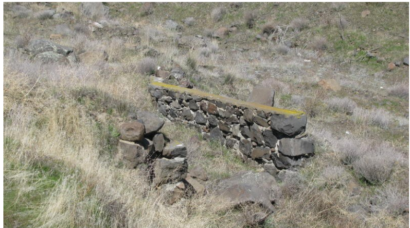
Bridge abutment on old wagon road to Hover
